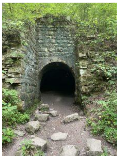
Richland Mine Entrance
